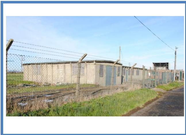
Figure 23: Remains of Sawtry Camp - Original POW Camp Prefabricated Concrete Buildings - May 2019 Copyright: ©2019 Martin J Richards BA(Hons) ARPS (Systonimages.co.uk)
